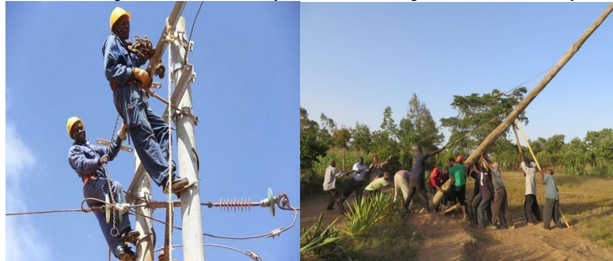
Plate 1B: showing installation of electricity Plate 1C: showing installation of electricity
