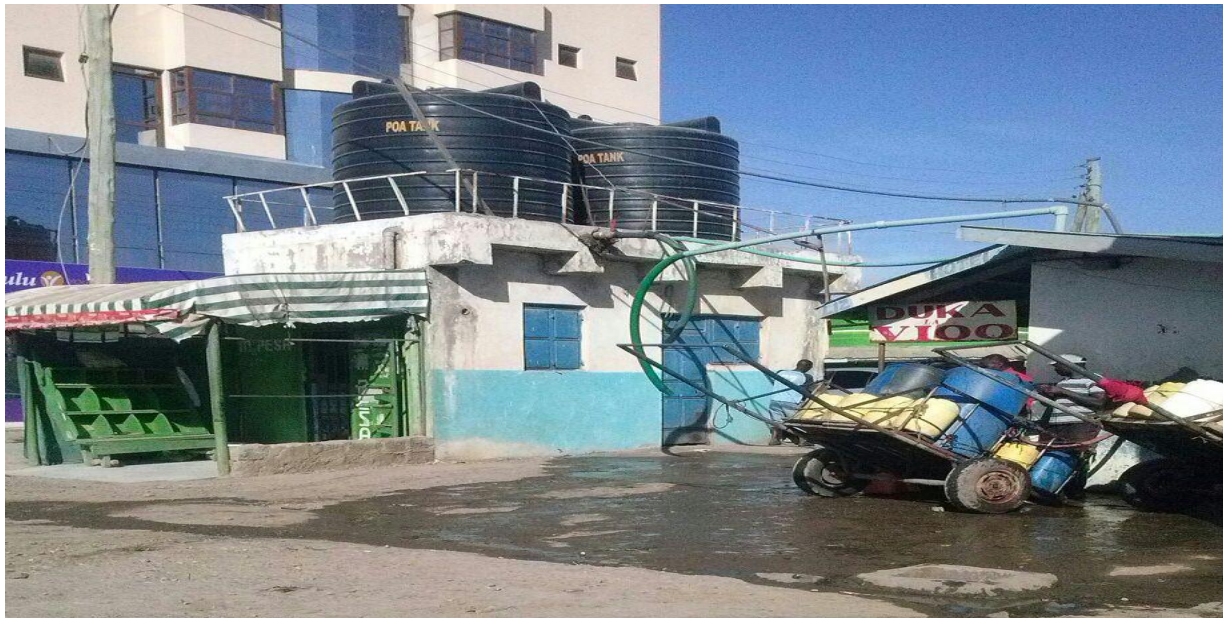
Source: Author Plate 4.4 PCEA water project in Kitengela
