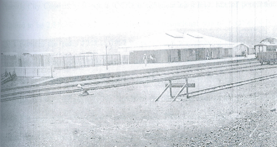
Plate 3. 1: The first railway station in Kisumu in 1901 Source: Town Planning Department-CCK
