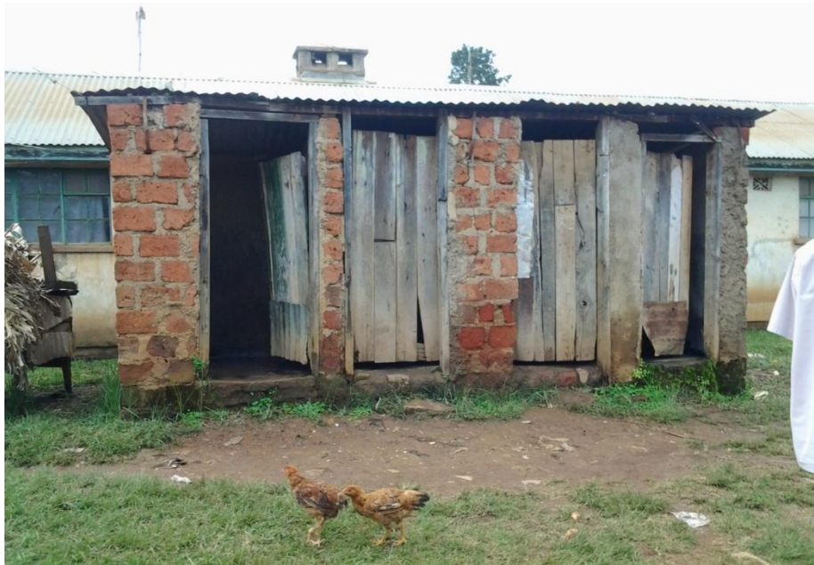
Figure 4.3: Plate 3: Prison latrines in one of the prisons
